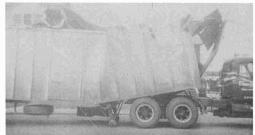
"Can't you read the 'Low Clearance' sign?" A truck damaged by the viaduct's low clearance.
